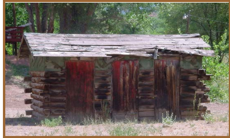
Historic Sanitation Structure
