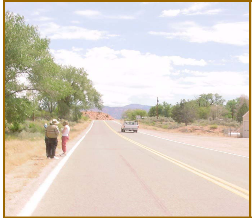
Highway 141 – North view from Dolores River Bridge
