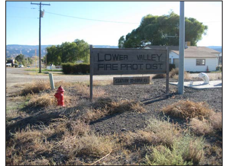
Photo 1: Loma Fire Substation
