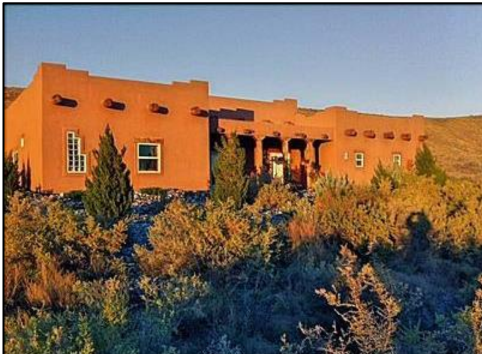
Figure C.59. Kannah Creek home.
