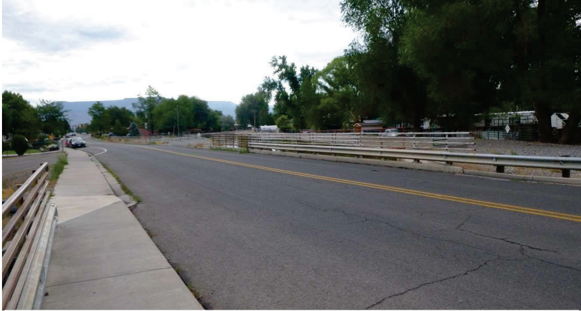
Figure 61: Project Area overview at Grand Valley Canal
