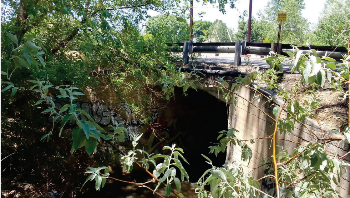
Figure 64: Lewis Wash culvert at Orchard Avenue, looking northwest
