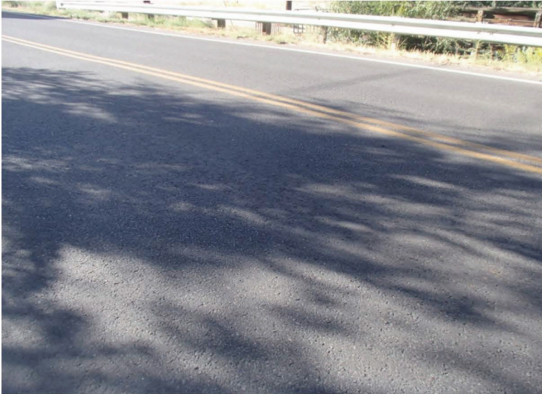
View of deck
