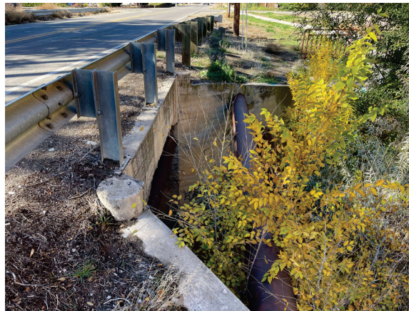
Photo 1 – Upstream End of Existing Culvert Structure at e 1/2 Road
