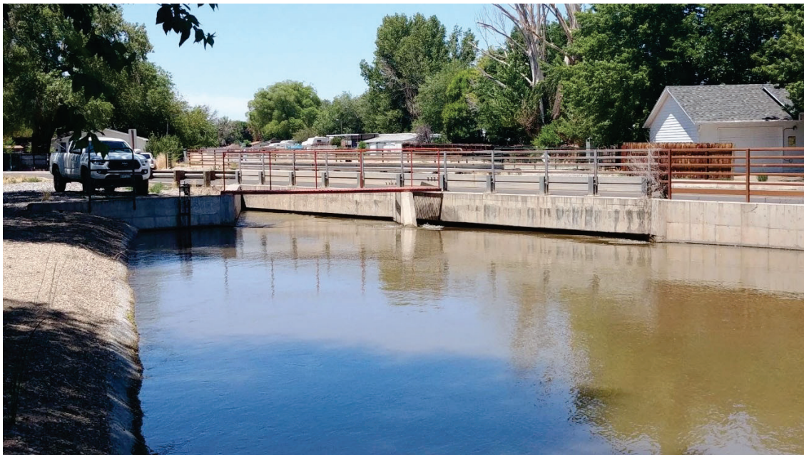
Figure 63: Grand Valley Canal Box culvert at Orchard Avenue, looking west-northwest
