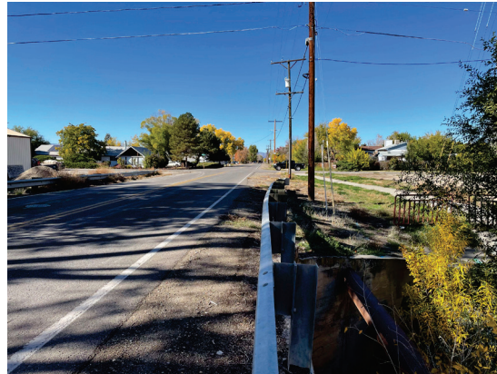
Photo 2 – Orchard Avenue – Looking West at Upstream End of Existing CBC
