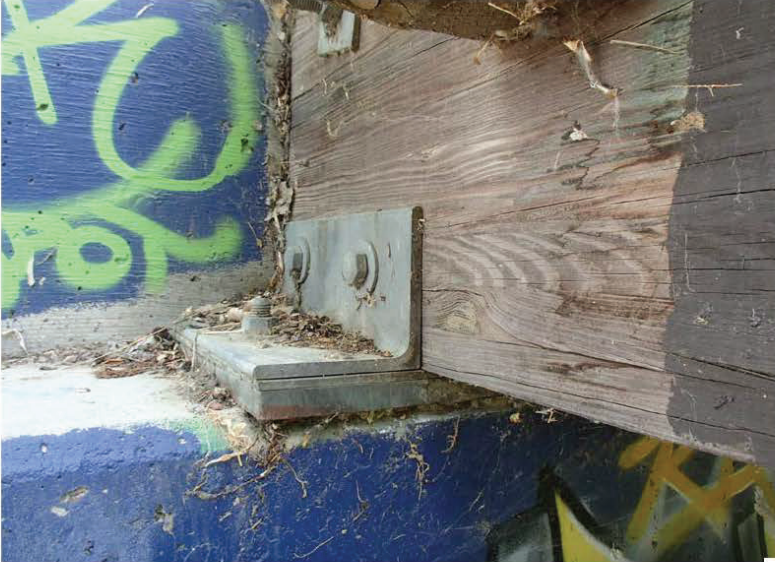
Typical bearing condition
