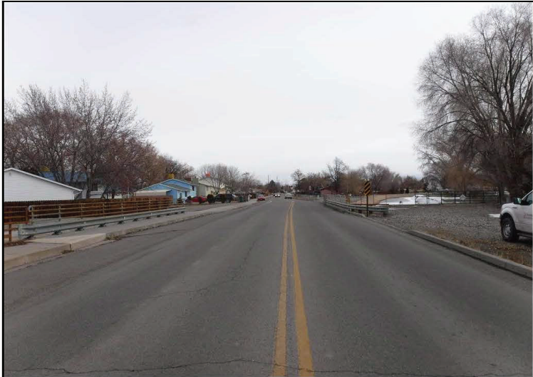
Roadway looking east
