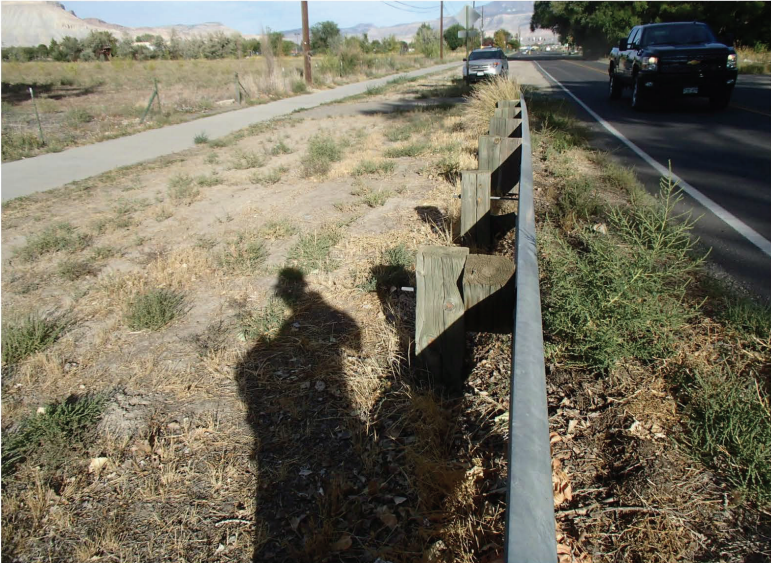
Twisted blocks on northeast approach rail
