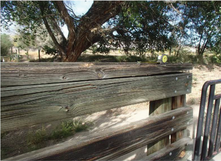
Cracked and weathered rail at northwest corner
