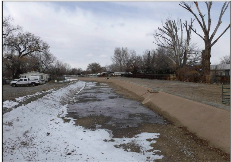
Channel looking downstream
