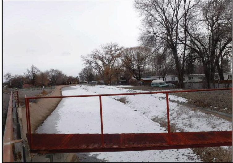
Channel looking upstream
